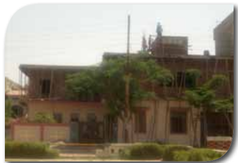
The Karishma Girls Home 2nd floor under construction - Agra, India.
